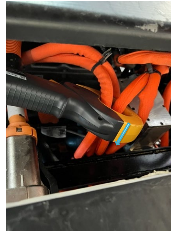
Figure 13. Clamp on the front cables
