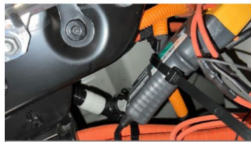
DCAC & HVAC – 200A
